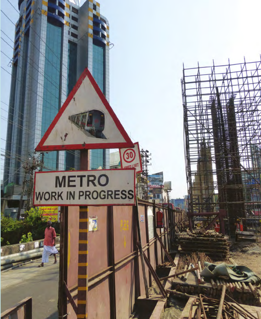
Figure 21 : Metro under construction in Kochi, Kerala State
