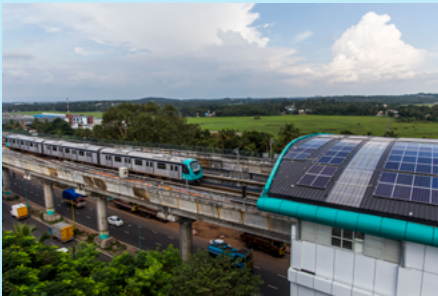
15. Solar panels installed on the roof of metro stations © Prashanth Vishwanathan/AFD
