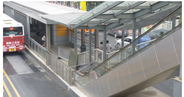
Figure 12: Escalators not working at a BRT station. Photo by Heather Allen.
