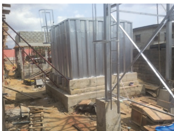
FIGURE 12: WATER TANK IN PROGRESS
