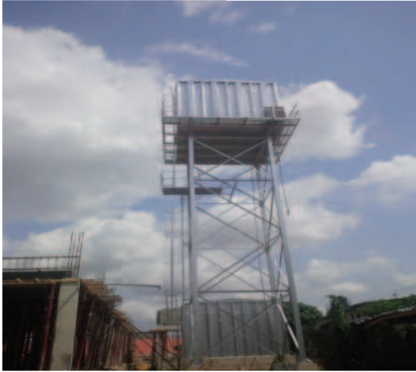
FIGURE 16: CABLE TRENCH DUCT AND WATER TANKS
