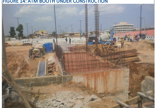
FIGURE 14: ATM BOOTH UNDER CONSTRUCTION
