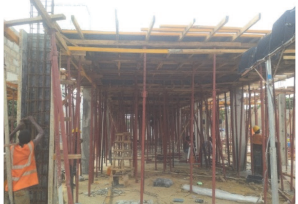
Figure 13: TERMINAL BUILDING CONSTRUCTION IN PROGRESS
