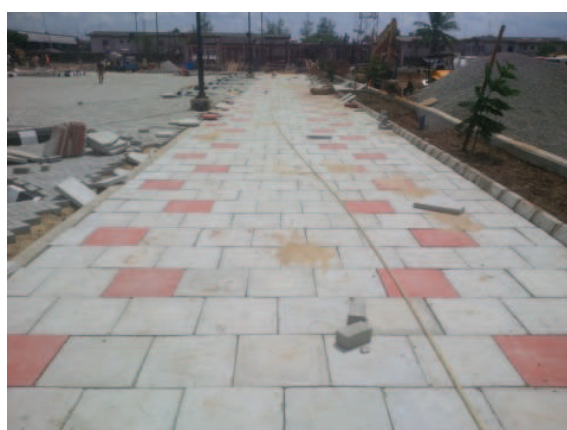
FIGURE 15: PAVEMENTS NEARING COMPLETION
