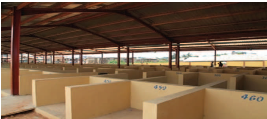
FIGURE 25: MARKET STALLS CONSTRUCTED BY LAMATA AT OLUWO ODUKAN FOR PAPs
