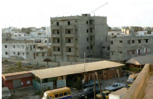
This infill building development in Dakar, Senegal, densifies the existing urban footprint and is accessible by local transit.
