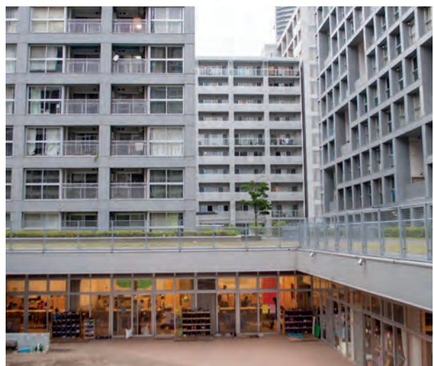
This ground floor kindergarten facility at Shinanome, Tokyo, Japan, is conveniently accessible to the parents and children living above and around.
