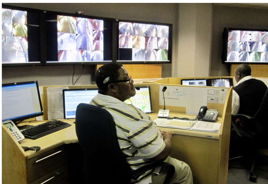
Figure 12. Control centre in Johannesburg, South Africa.
