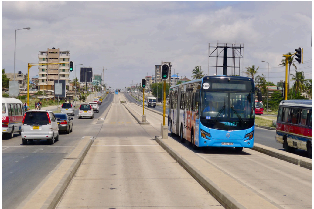
Figure 14. BRT corridor in Dar es Salaam, Tanzania.
