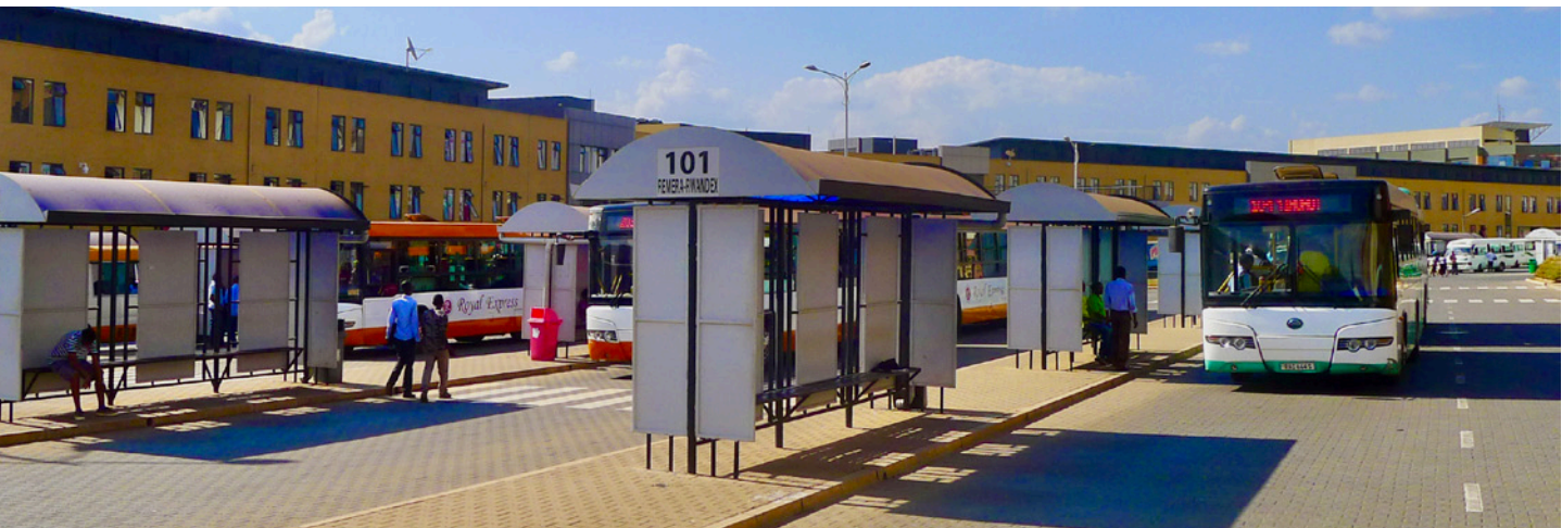
Figure 16. Bus terminal in Kigali, Rwanda.
