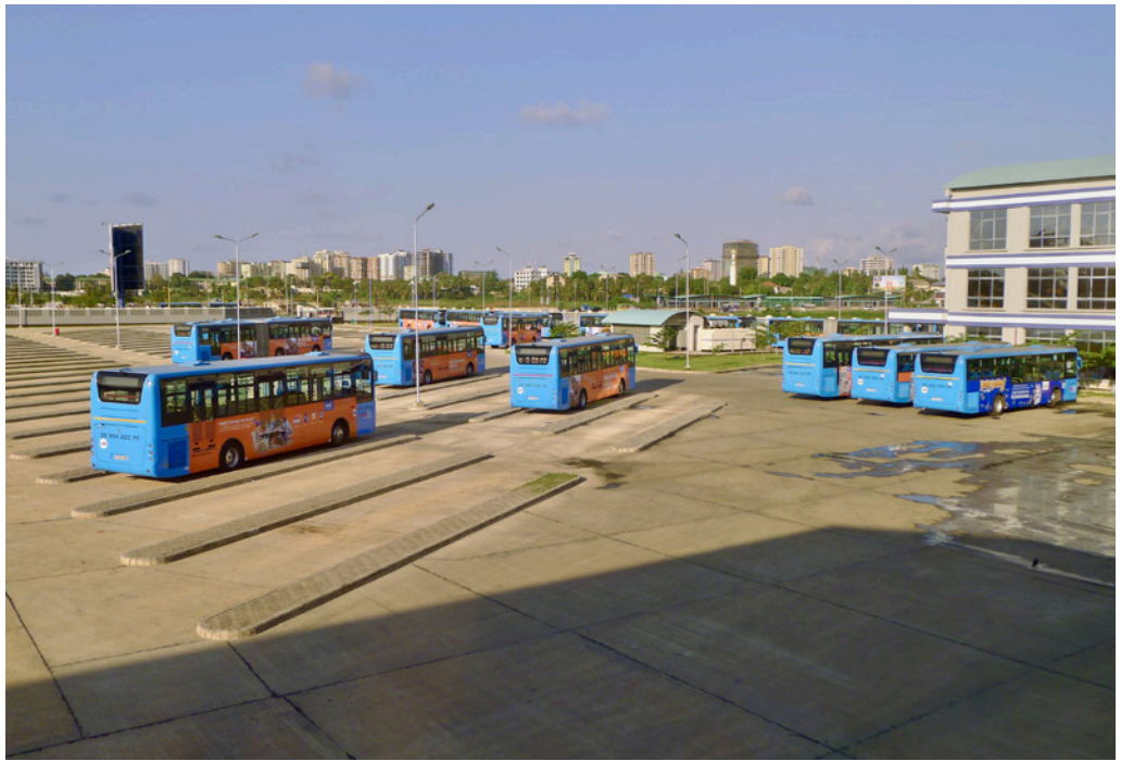
Figure 25. Bus depot in Dar es Salaam, Tanzania.
