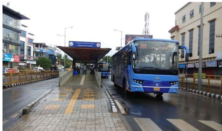
Well developed PT System
