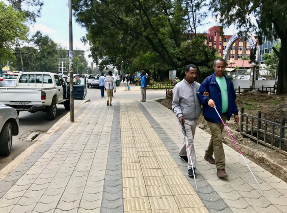
Figure 17. Footpath in Addis Ababa.
