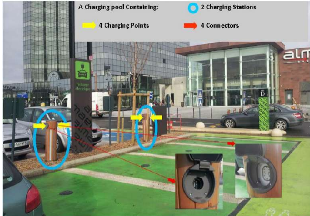
Figure 1.1: A charging pool with multiple charging stations and charging points (NEA, 2019)
