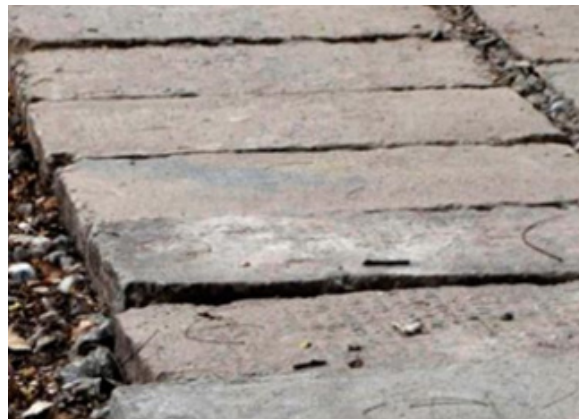
Storm water drains used as footpaths
