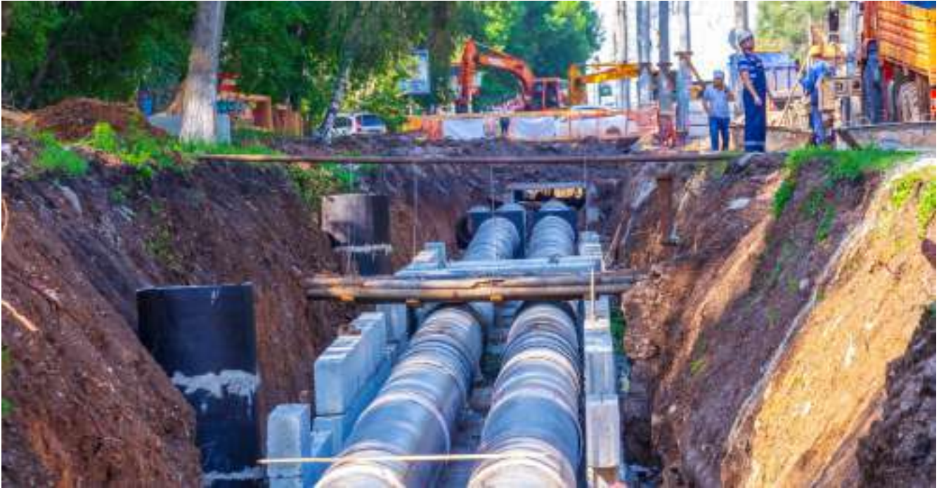
Repair work in the city to replace water pipes in the city of Samara, Russia © Shutterstock
