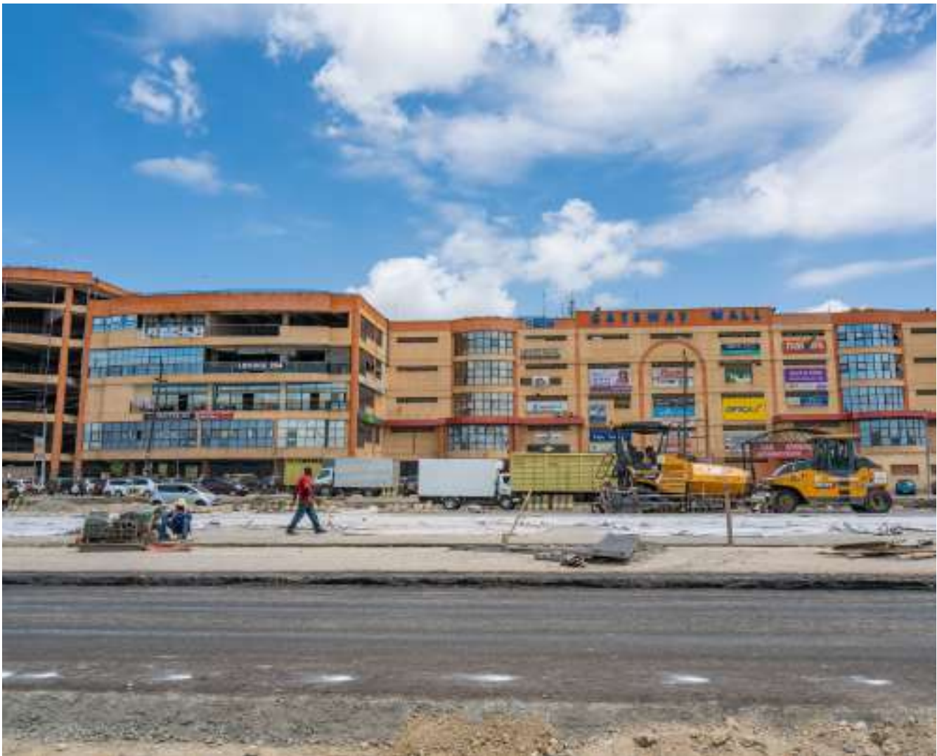
A Road under construction in Nairobi, Kenya. © NoyanYalcin/Shutterstock
