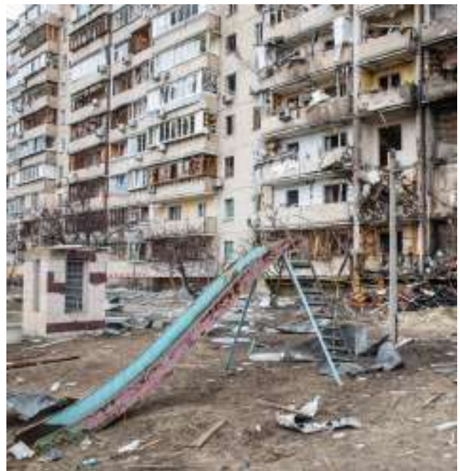
Damaged residential building, Kyiv, Ukraine © Drop of Light/Shutterstock
