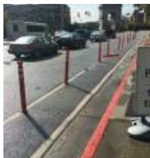
Flexible bollards delineate an interim bike lane.
