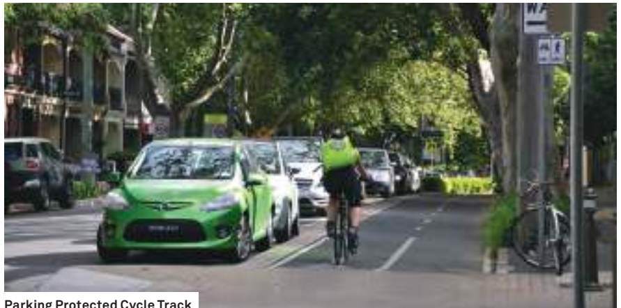
Parking Protected Cycle Track
