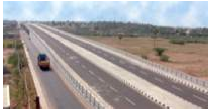
Figure 5.103: Raised median on dual carriageway.
