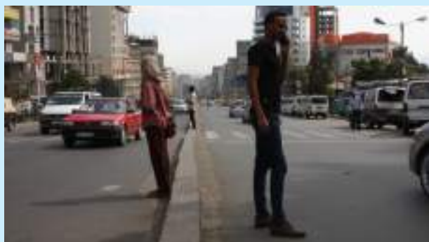
Figure 5.117: Narrow unsafe median
