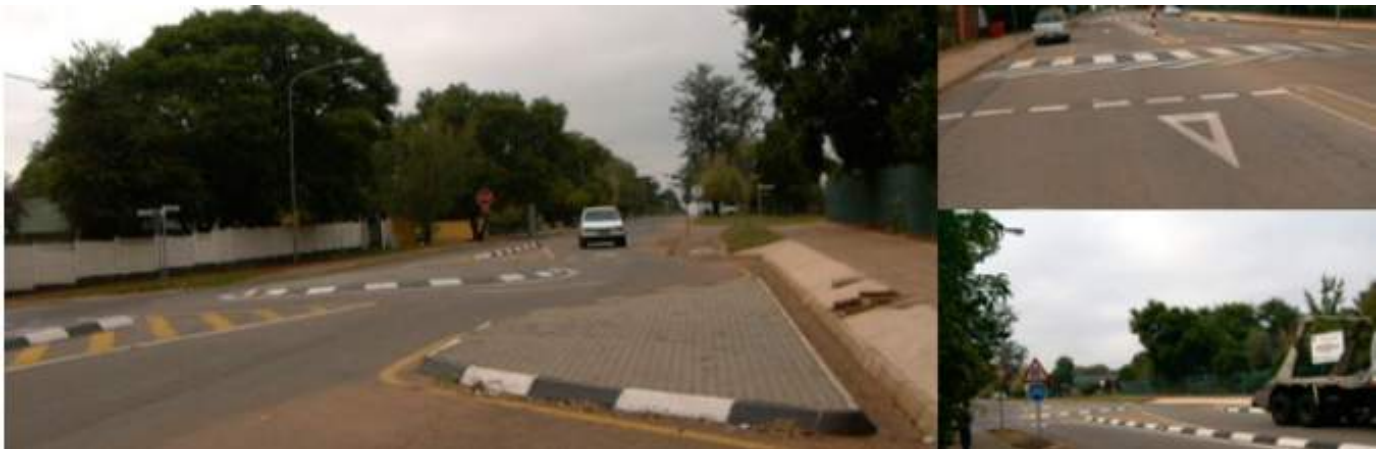
Figure 3.11: Use of mixed traffic calming infrastructure—narrowing, speed humps, and delineators
