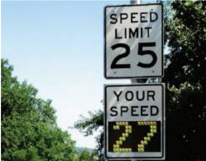
Figure 3.7: Speed feedback sign.
