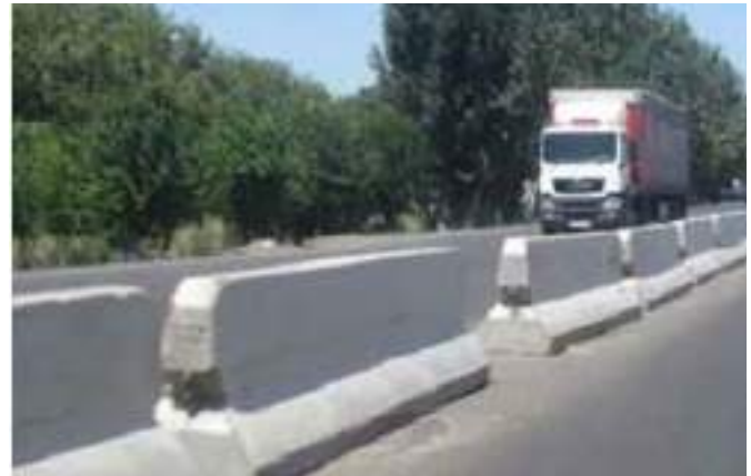
Figure 5.69: Individual concrete blocks.
