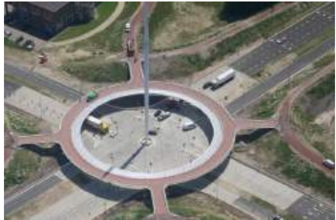
Figure 4.45: Floating roundabout for cyclists—Netherlands.
