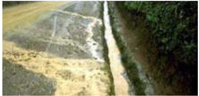
Figure 5.143: Armor ditches with vegetation, rock, masonry, or concrete to resist ditch erosion.
