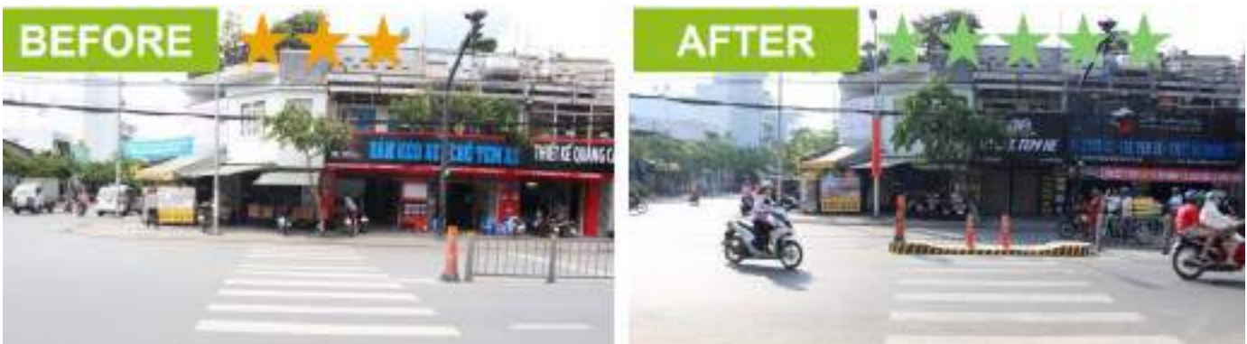
Figure 4.28: Installing pedestrian refuge—Vietnam.
