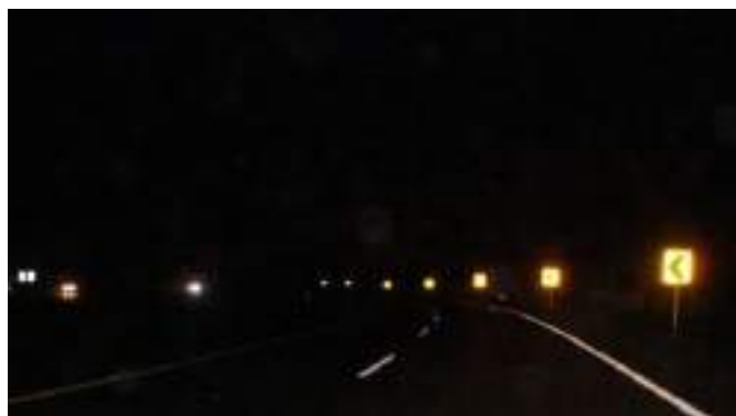
Figure 5.25: Chevron alignment signs providing good night-time visibility.
