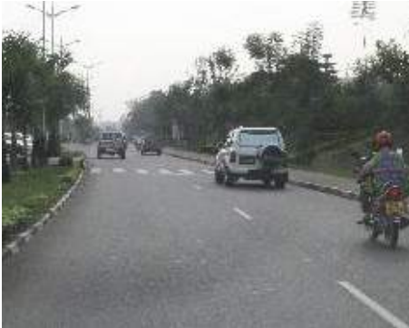
Figure 4.20: Well defined at-grade crossing—Rwanda.
