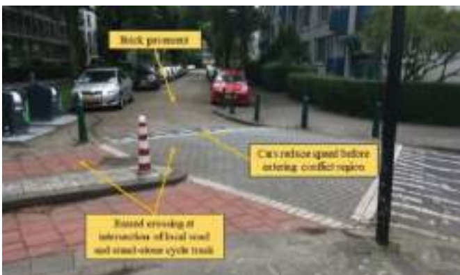
Figure 6.50: Raised intersection with different pavement pattern.
