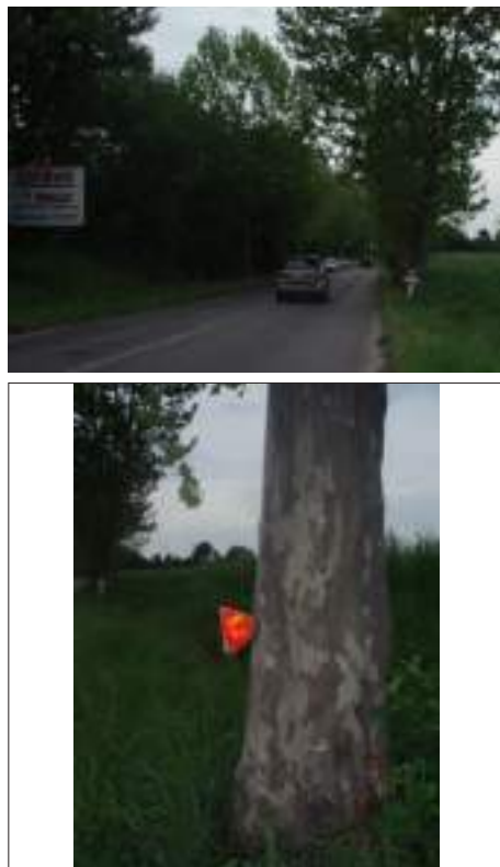
Figure 5.78: Roadside tree delineated but inconspicuous—Italy.
