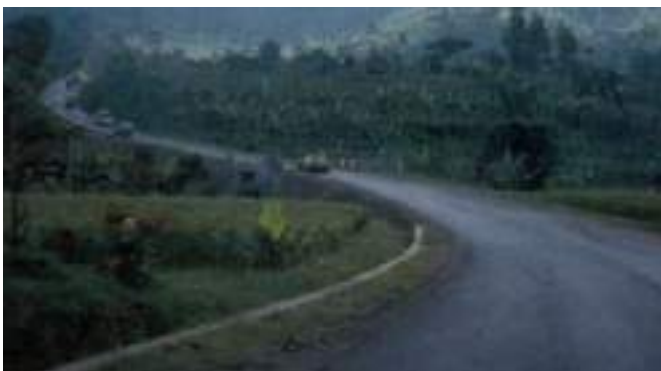
Figure 5.22: Example of good combination of horizontal and vertical curvature providing good visibility.
