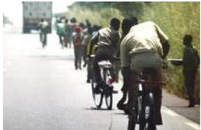
Figure 5.9: Narrow shoulders resulting in increased risks for cyclists on the travelled way
