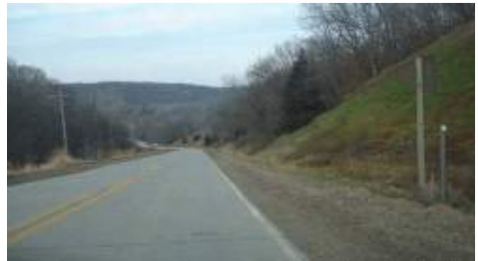
Figure 5.19: Hazardous combination of horizontal curve at the base of a steep upgrade.
