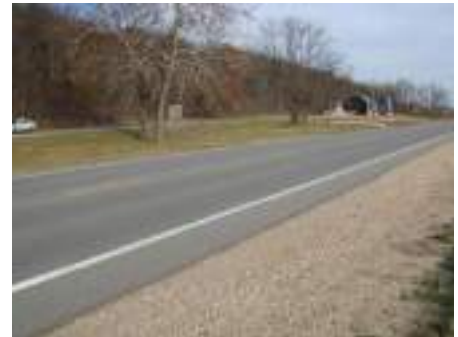
Figure 5.8: Partially-paved or composite shoulder
