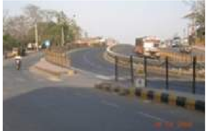
Figure 5.113: Use of nonstandard median type and unsafe median opening on a high-speed road.
