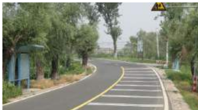
Figure 5.24: Transverse lines at the entrance of curve in China.
