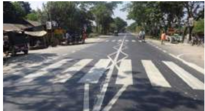
Figure 3.55: Well-maintained road with clear road markings—India.
