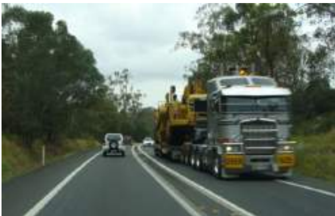
Figure 5.29: Wide centerline with median rumble strips on curve in Australia.
