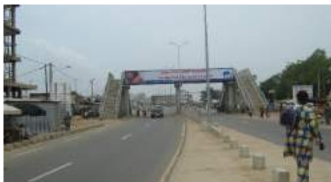
Figure 3.39: Opaque apron on footbridge may deter pedestrians from using the facility due to security concerns
