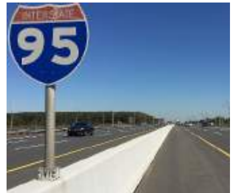
Figure 5.82: Rigid (F-profile) barrier.
