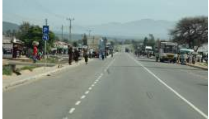
Figure 3.28: Separated roadside market space with parking, Dar es Salam corridor between Morogoro and Mafinga, Tanzania.
