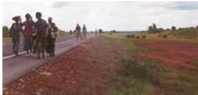
Figure 5.141: Earth excavated drainage in Malawi.
