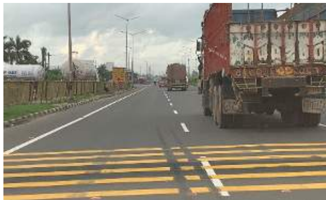
Figure 3.4: Rumble strips on highways.
