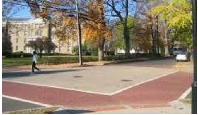
Figure 6.49: Raised intersection with colored pavement.
