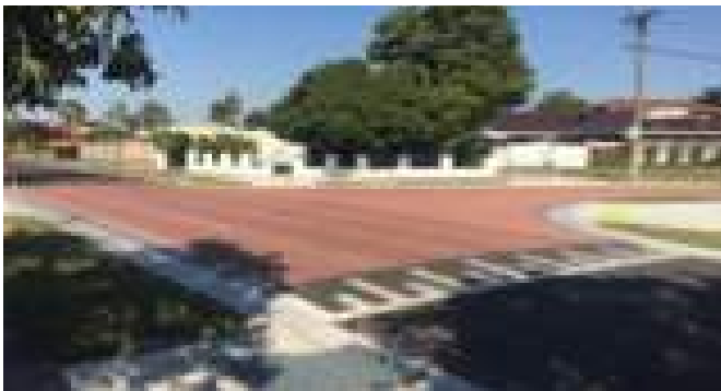
Figure 6.57: Colored, raised intersection with line markings.
