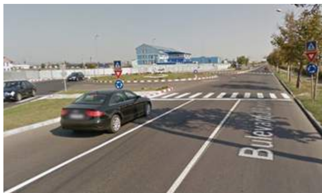
Figure 6.31: Dangerous roundabout design in Romania, where the main road has no deflection.
