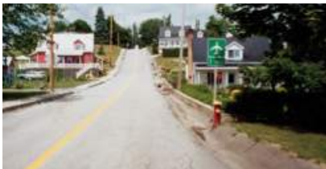
Figure 5.138: Hazardous drainage facility on a narrow and hilly road.
