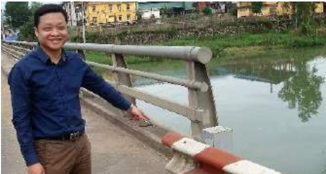
Figure 5.87: The exposed end of the guardrail can spear through an impacting vehicle.
