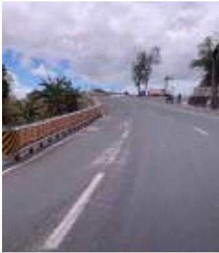
Figure 5.91: Fully re-directive crash cushion—Philippines.
