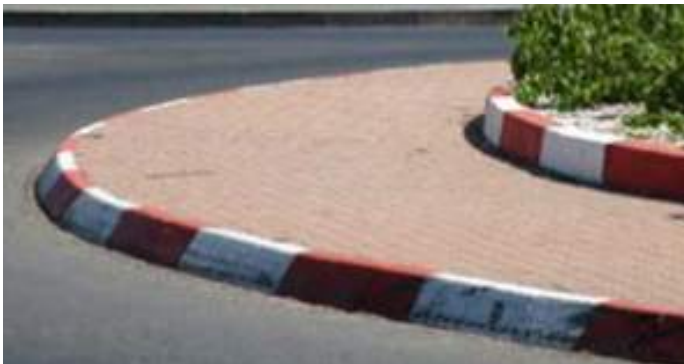
Figure 6.38: Truck apron not serving the purpose of design in South Africa (too high apron to ride on for larger trucks and too low to block riding on passenger cars).
