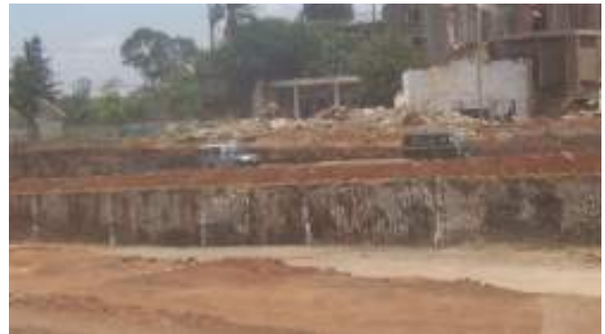
Figure 3.49: Major excavation with no protection or segregation of work zone and general traffic—Kenya.
