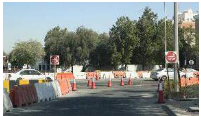
Figure 3.47: Well signed and guarded work zone—Abu Dhabi.
