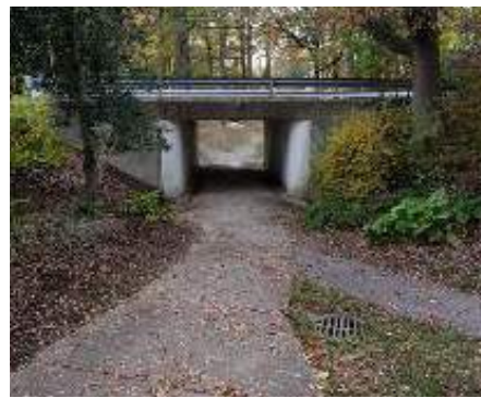
Figure 4.16: Grade separated underpass—US.
