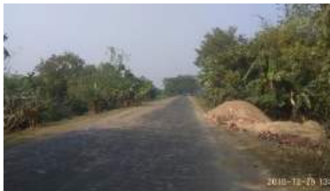
Figure 5.71: Stacked materials by the roadside. These are a particular hazard to two or three wheelers especially at night.
