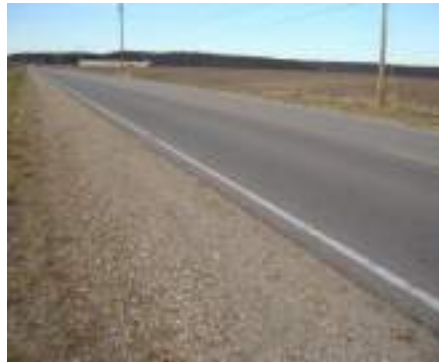
Figure 5.7: Unpaved gravel shoulder.
