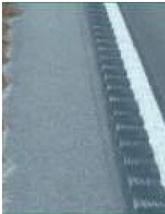
Figure 5.33: Edge line rumble stripes by milling of road.
