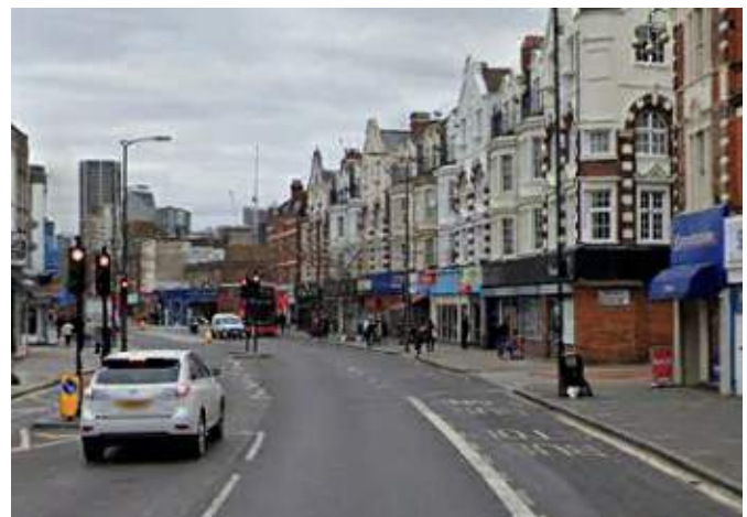
Figure 4.64: Bus lane and priority signal—UK.
