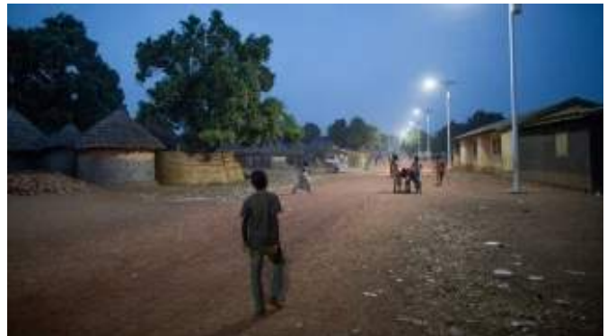
Figure 5.168: Solar powered streetlights.,
