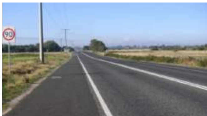
Figure 5.13: Wide sealed shoulder.
