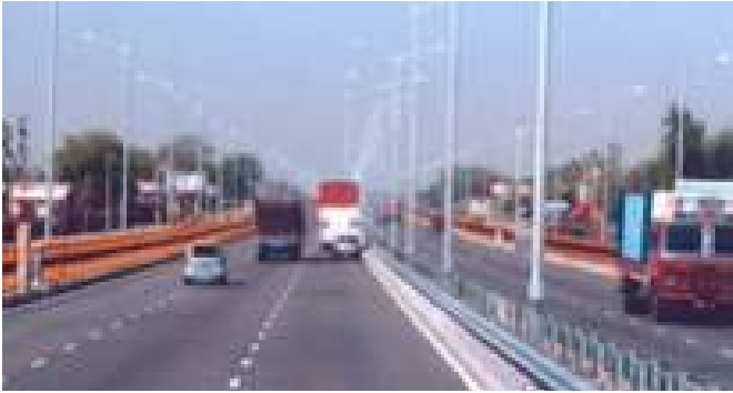
Figure 5.102: Semi-rigid median barrier on expressway.
