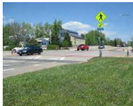
Figure 6.53: Raised intersection with crossing sign.
