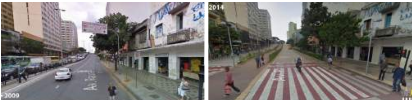
Figure 5.4: Example of a road diet in Brazil showing reduction in the number of lanes from three each way in 2009 to two each way in 2014, with the addition of a wide median footpath and cycle lanes.
