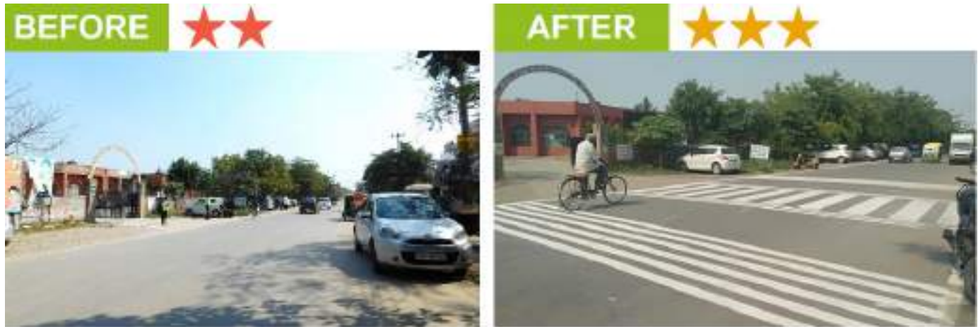
Figure 4.47: Installing crossings with advance cycle stopline—India.
