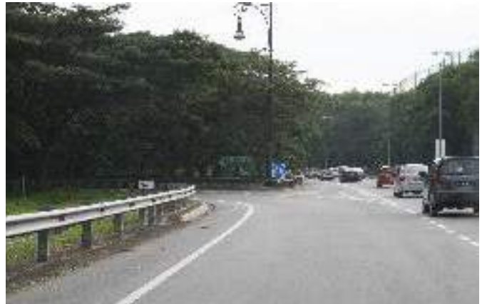
Figure 6.78: Deceleration lane approach tight exit radius—Brunei.
