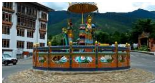
Figure 6.33: Decorated roundabout obscuring driver's sight in Bhutan
