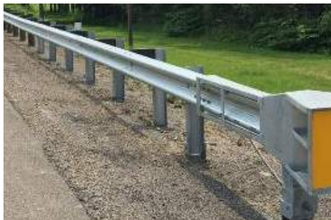
Figure 4.53: Typical metal barrier.
