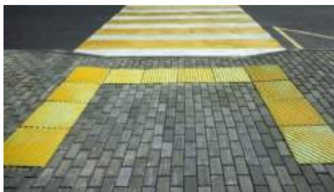
Figure 5.155: Dropped curb at both ends of pedestrian crossing with tactile paving surface.
