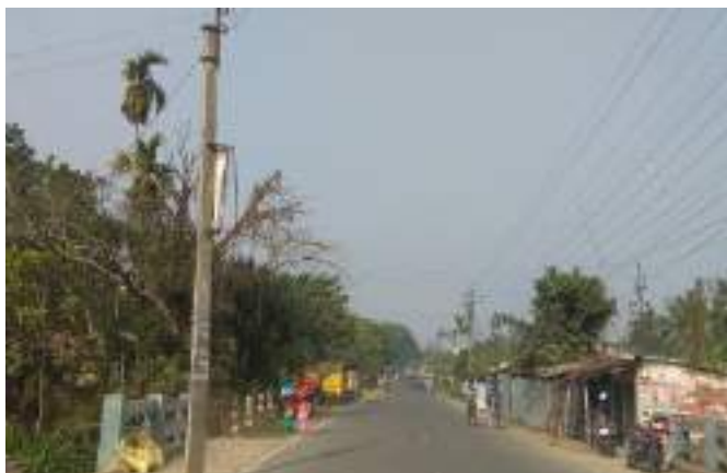
Figure 5.70: Rigid mast on shoulder.
