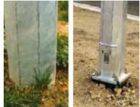
Figure 5.76: Impact-absorbing lighting columns suitable for low-speed
