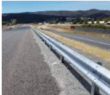
Figure 5.81: Semi-rigid barrier (W-beam).
