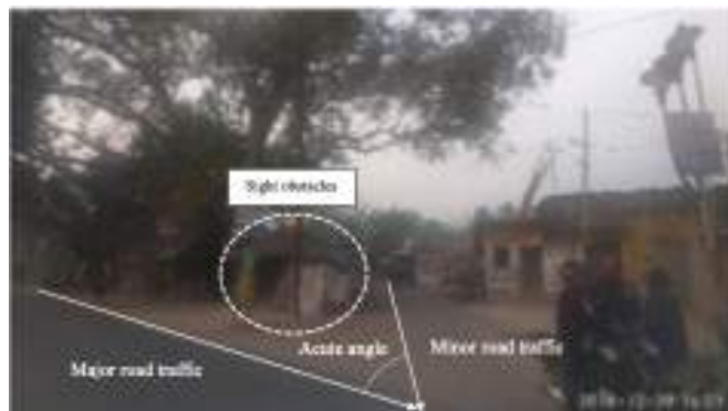
Figure 6.1: Uncontrolled Y-intersection in India.
