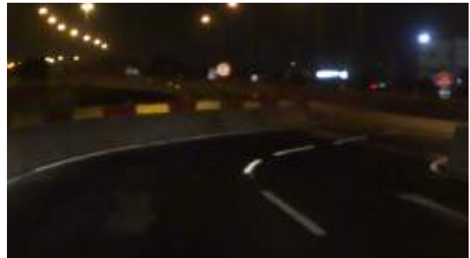
Figure 5.166: Line markings illuminated by retroreflecting material.
