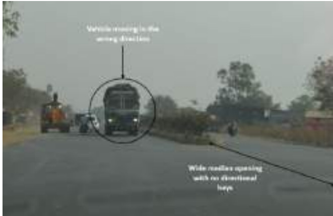
Figure 5.112: Unsafe median opening leading to contraflow.
