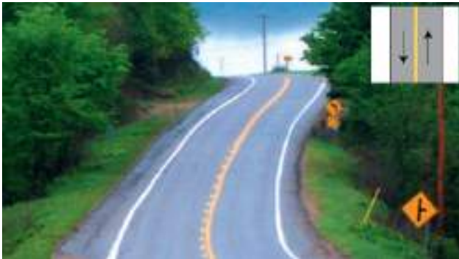
Figure 5.27: Horizontal curve at the base of a steep downgrade with advance warning sign.
