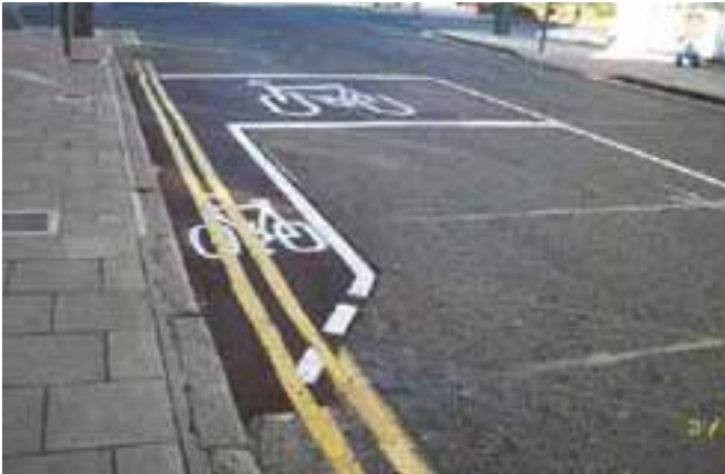
Figure 4.42: Advance cycle stopline (bike box) with contraflow cycle lane.
