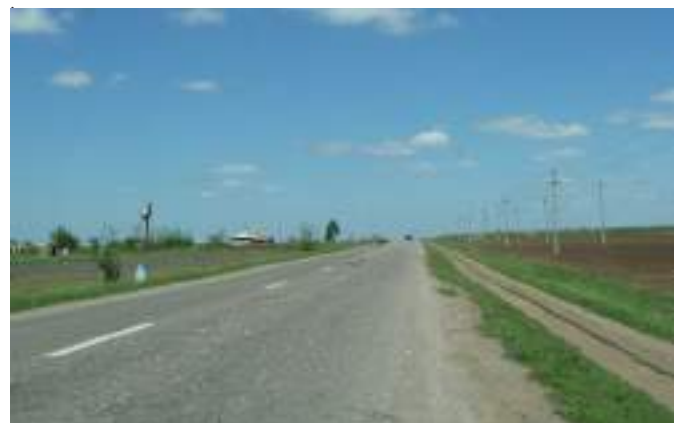
Figure 3.32: Moldova—service road for slow vehicles
