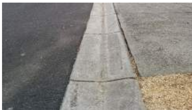
Figure 5.148: Sloping curb providing access to driveway.
