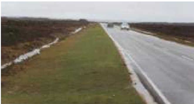
Figure 5.144: Safely widened shoulder and drainage.
