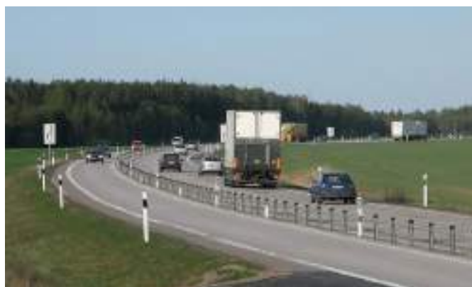
Figure 5.59: 2+1 highway with flexible barrier.
