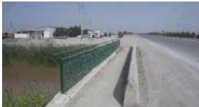
Figure 5.86: Light-gauge rails with concrete curbs.
