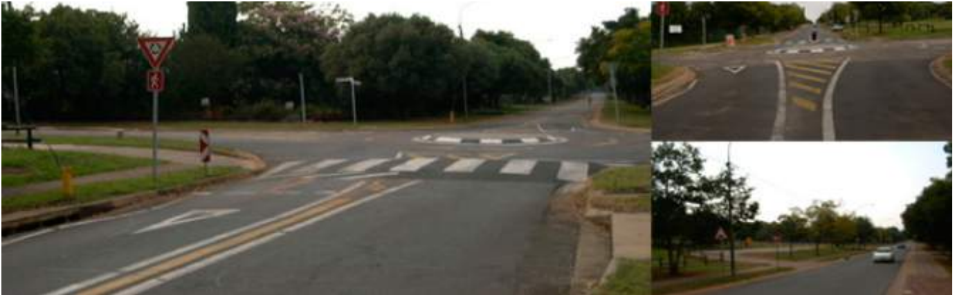
Figure 3.10: Raised pedestrian crossing and mini circle
