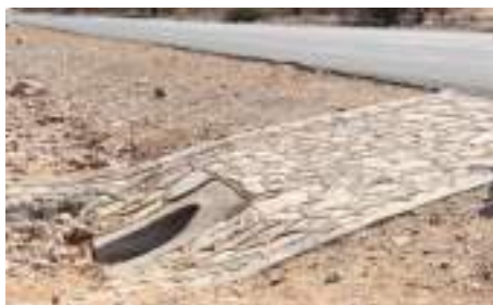
Figure 5.132: Typical extended culvert and revised headwall design.
