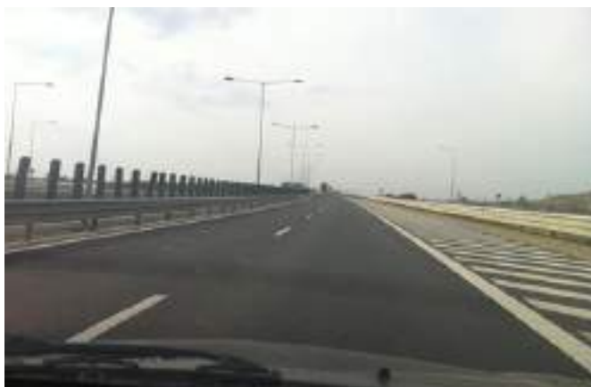
Figure 5.116: Anti-glare barrier on top of median.
