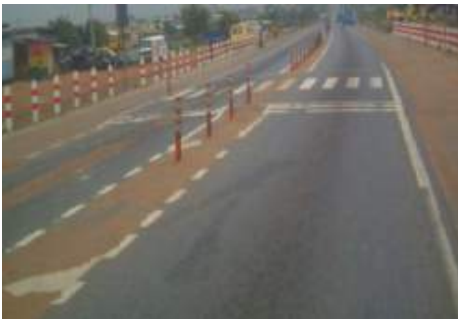
Figure 3.2: Carriageway narrowing, delineators, and speed humps.
