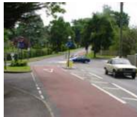
Figure 5.125: High friction surface (colored) applied on the approach to a mini roundabout.
