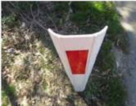
Figure 5.74: Lightweight guidepost that is forgiving.
