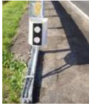
Figure 5.92: Fully re-directive terminal, flared or tangential.
