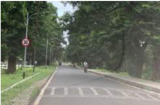
Figure 3.33: Speed sign and speed hump for gateway treatment—India.
