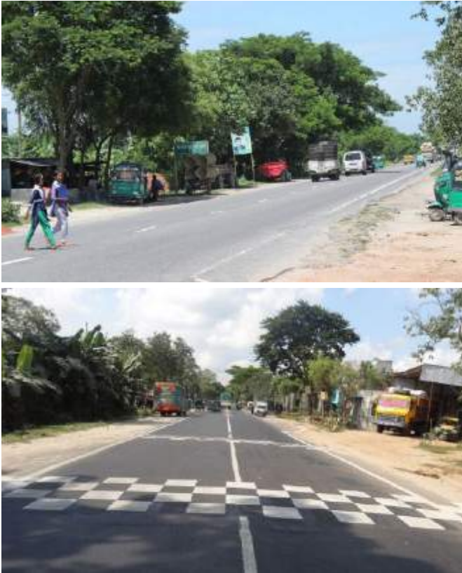
Figure 3.14: Installing speed table with checker marking. Left: before the intervention; Right: After the intervention.
