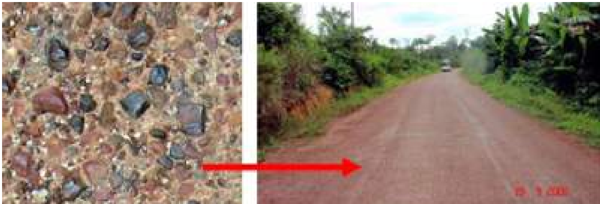
Figure 5.122: Otta seal surfacing on low volume road in good condition with satisfactory results. (left image: close-up of the otta seal surfacing).
