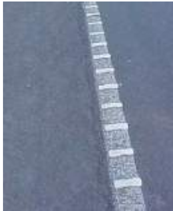
Figure 5.32: Edge line rumble stripes by adding ribs.
