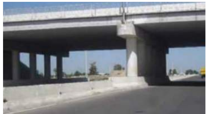
Figure 5.77: Shielded piers with rigid barriers. An appropriate end treatment (cushions/impact attenuators) should also be applied on barrier systems.
