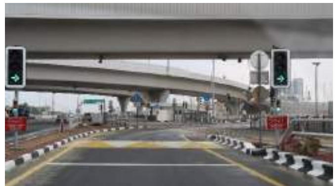
Figure 6.86: Automatic signal controlled crossing—Dubai tram.
