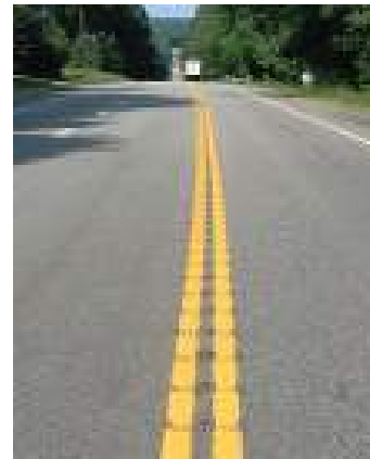
Figure 5.34: Centerline rumble stripes by milling of road.
