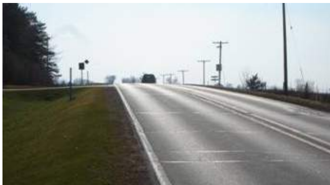
Figure 5.40: Reduction in sight distance at a crest vertical curve.
