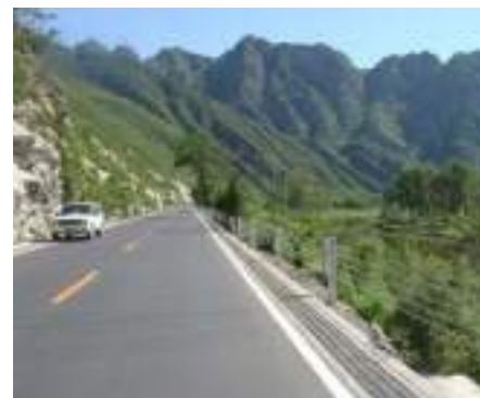
Figure 5.37: Cable barrier on tangent section.
