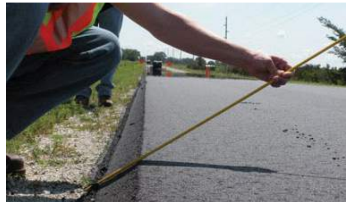
Figure 5.30: Safety edge. After installing the safety edge, the unpaved material adjacent to the edge should be graded flush with the top of the pavement.
