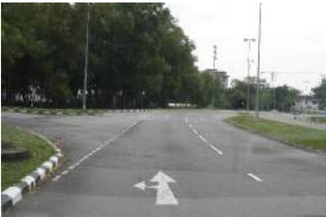
Figure 6.75: Urban LILO Brunei with insufficient space for safe lane change to offside right turn.
