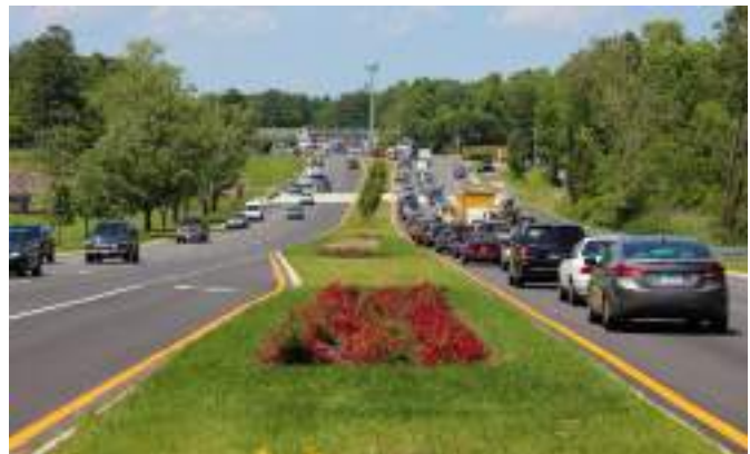
Figure 5.115: Raised median on carriageway.
