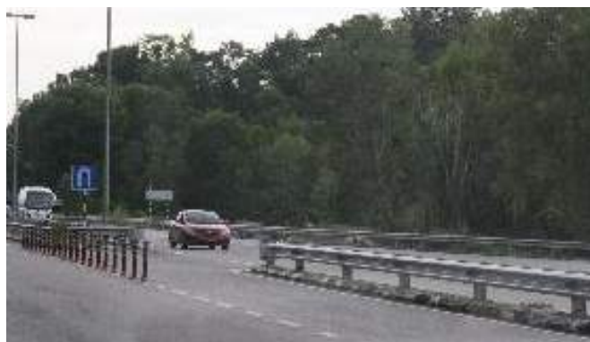
Figure 6.81: Additional barrier to offside diverge—Brunei—to control entry and turning area beyond far carriageway for ALL vehicles, adding additional merge after crossing opposing traffic.
