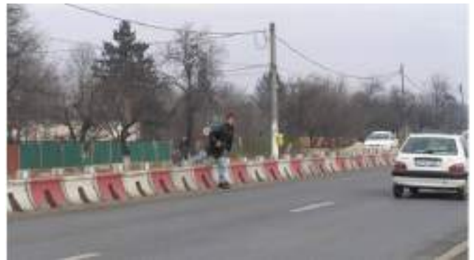
Figure 3.26 Poorly designed median for no crossing location—Romania.
