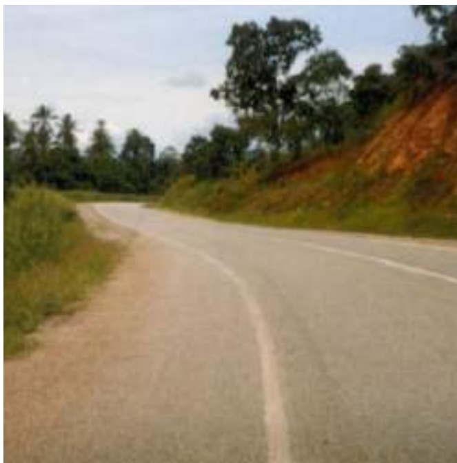
Figure 5.38: Example of introduced superelevation on curve
