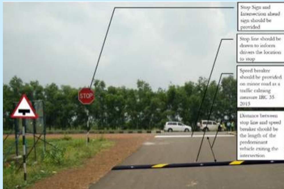
Figure 6.12: Minor road treatments—traffic calming and warning signs in India from minor road perspective.
