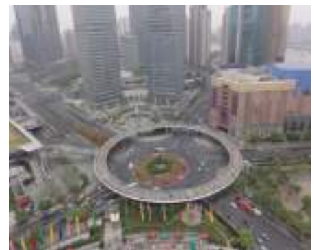
Figure 4.17: Well designed foot bridge—Shanghai.
