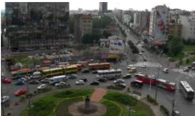
Figure 6.39: Roundabout (rotary) with improper lane alignment and width creating extra lanes in Serbia.
