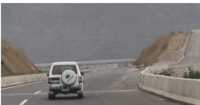
Figure 5.44: Escape ramp (under construction) in China.
