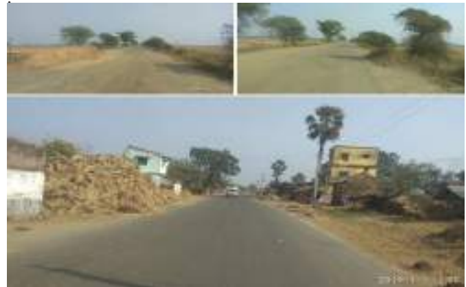
Figure 3.53: Stacked construction material unprotected or contained along the highway—India
