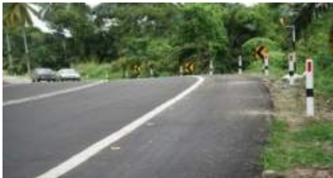
Figure 5.14: Wide, paved shoulder on curve.
