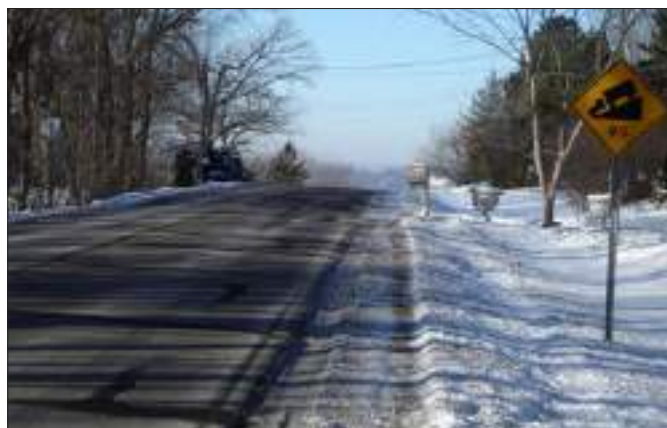
Figure 5.48: A steep grade warning sign along a road that appears to drop off in the distance.
