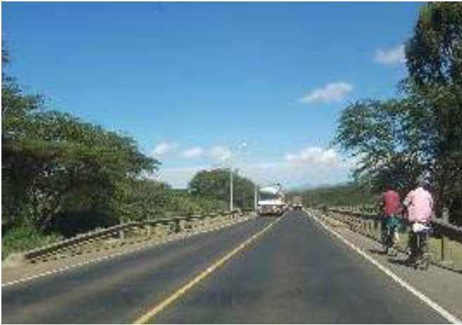
Figure 4.32: Cyclists using a narrow shoulder—Rwanda.
