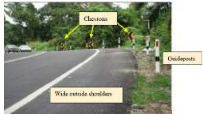
Figure 5.28: Example of curve improvement in Malaysia.
