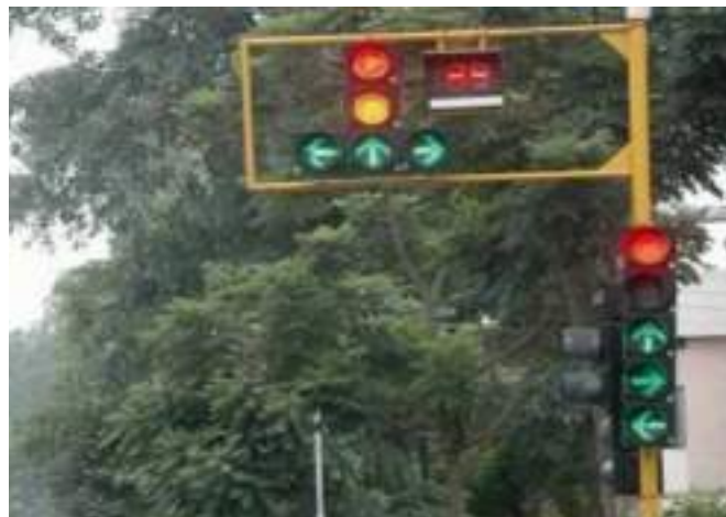
Figure 6.17: Traffic control signal for vehicles in India.
