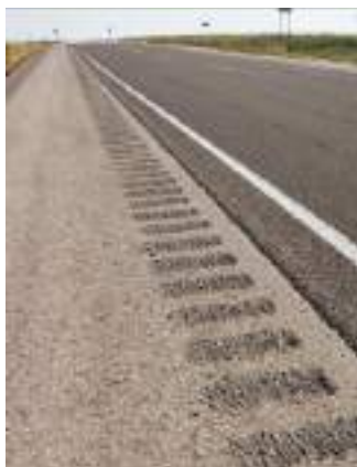
Figure 5.31: Shoulder rumble strips.
