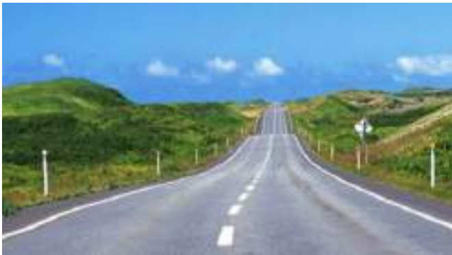
Figure 5.20: Poor alignment combination showing optical breaks caused by steep sag curves along horizontal tangent.
