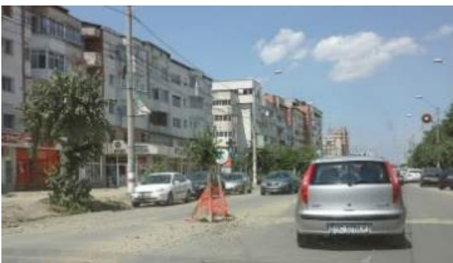
Figure 3.50: Construction with no protection or segregation of work zone and general traffic—Romania.
