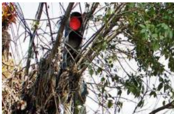
Figure 6.18: Signal hidden by the branches of a tree in Gurudwara, India; tree/branches must be removed or replace signal.
