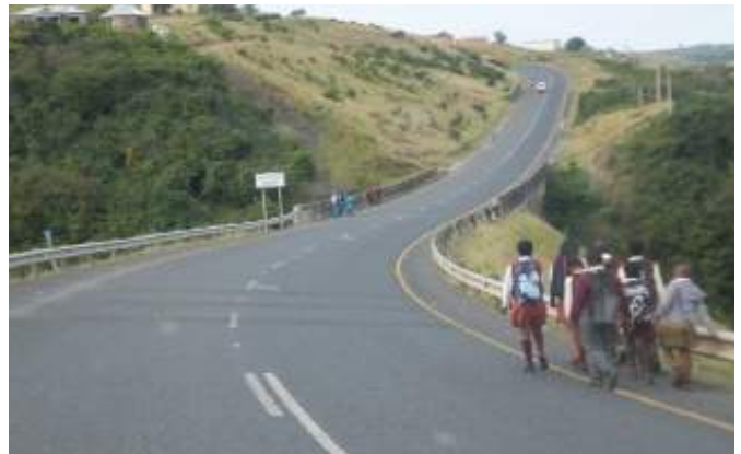
Figure 4.11: Unprotected footpath on rural national road.
