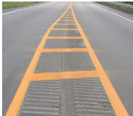
Figure 5.97: Flush median with rumble strips.
