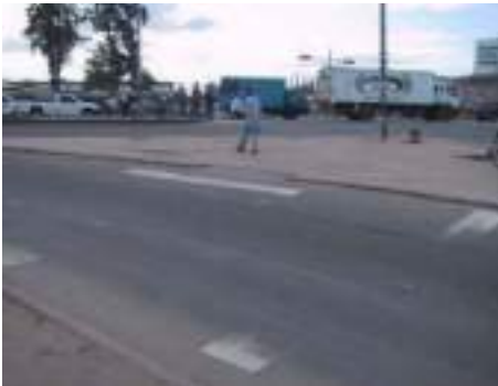
Figure 6.61: No marking slip lane in Tanzania.
