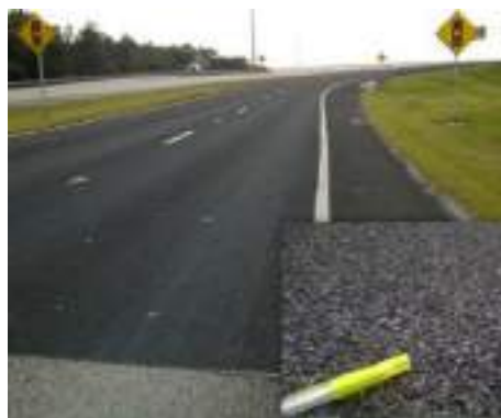
Figure 5.123: High friction surface treatment on high-risk curve.
