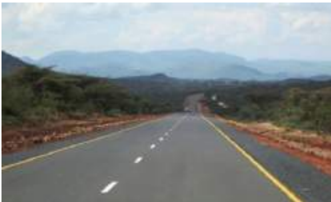
Figure 5.120: An asphalt road surface in good condition.
