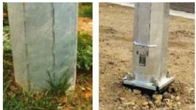
Figure 5.170: Impact-absorbing lighting columns suitable for low-speed environments with higher pedestrian activity and parking.
