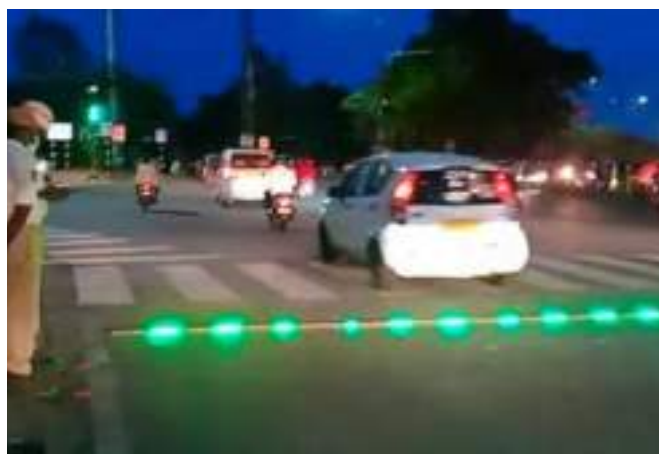
Figure 6.28: Pedestrian-cross-assistance devices (signals on cross walk) in Hyderabad, India.
