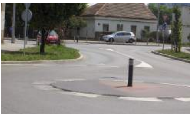
Figure 6.41: Mini-roundabout with noticeable pole—Zagreb, Croatia.
