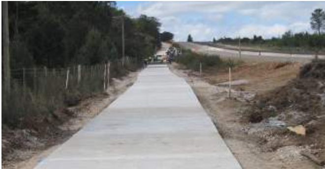
Figure 4.12: Segregated pedestrian/nonmotorized transport facility on rural road.
