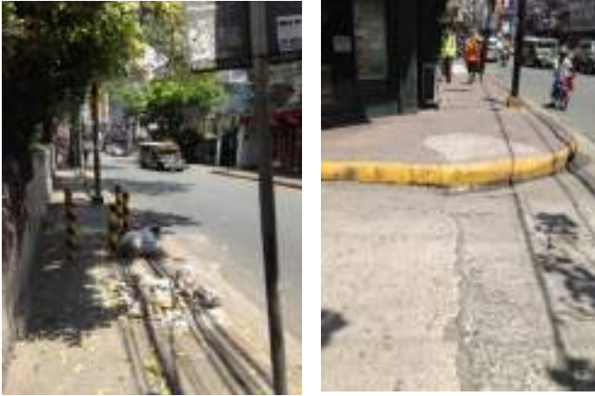
Figure 4.8: Obstructed footpath, and lack of drop curb in Manila.
