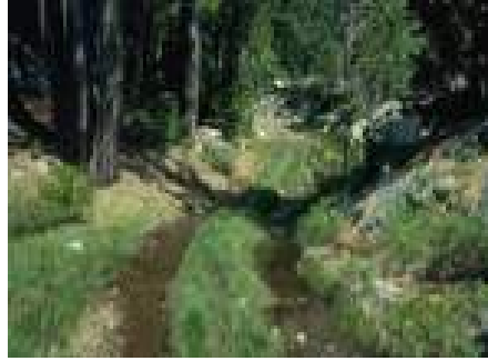
Figure 5.136: Poor road location with creek and hydrological connection to streams.
