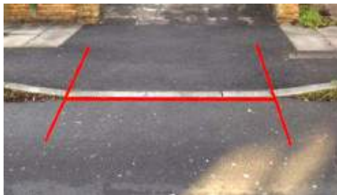
Figure 5.156: Dropped curb providing access to property.
