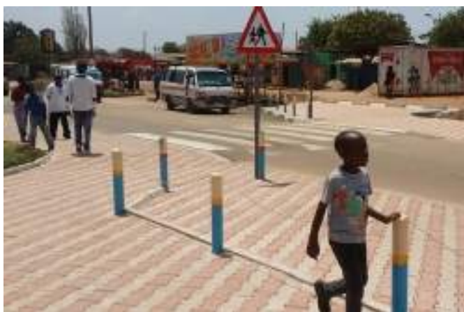
Figure 3.13: School children are protected by an elevated zebra crossing which is a traffic calming feature in itself.
