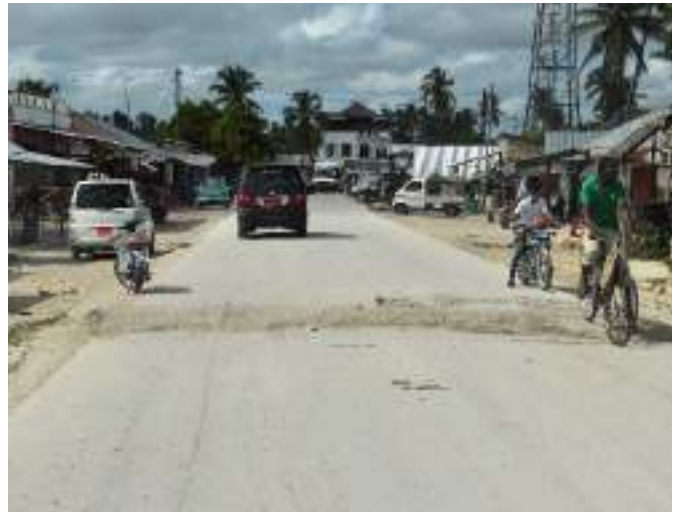
Figure 3.8: Unmarked ("invisible") speed hump—Zanzibar.
