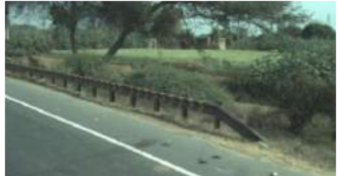
Figure 5.88: Unsafe ramped end of semi-rigid barrier that can launch an impacting vehicle.
