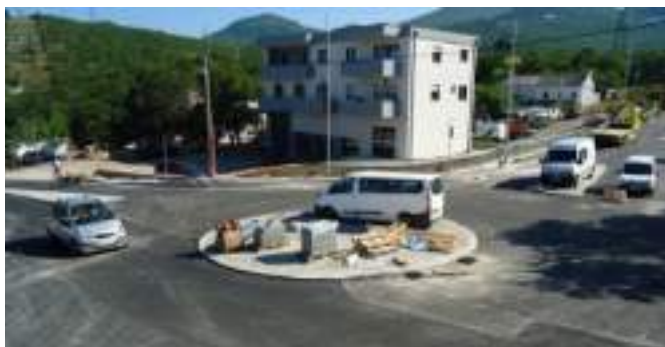
Figure 6.32: Vehicle ignoring flat roundabout in Croatia
