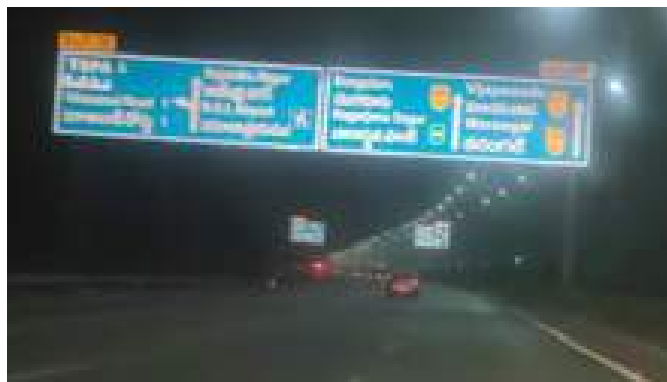
Figure 5.163: Expressway with interchange signs and lighting in Hyderabad, India.
