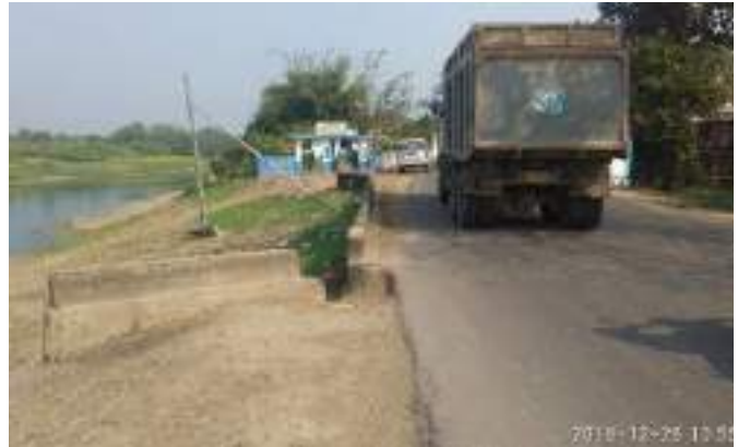
Figure 5.67: Unshielded water body with steep embankment.
