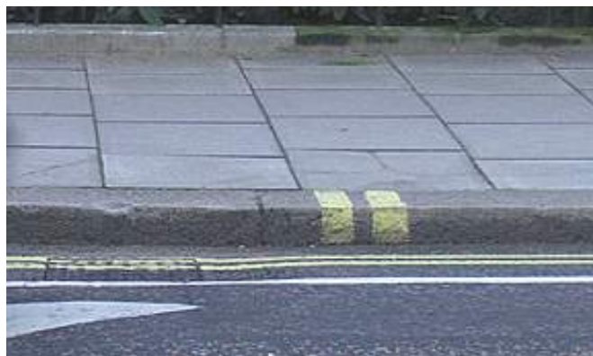
Figure 5.147: Concrete vertical curb.
