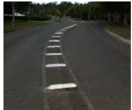
Figure 5.98: Median with pavement bars.
