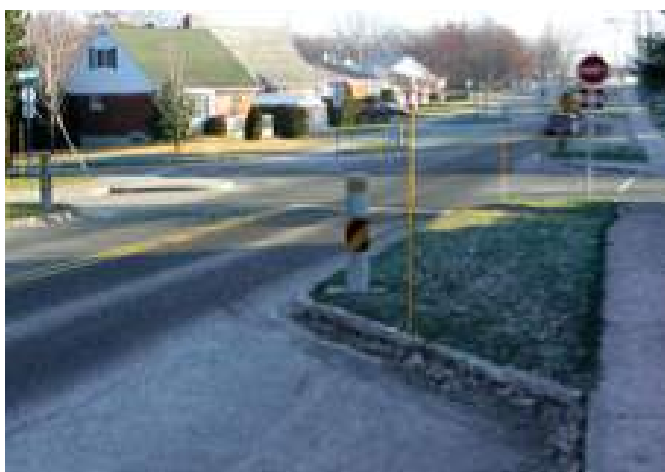
Figure 6.6: Stop signs with traffic calming measures at unsignalized intersection.
