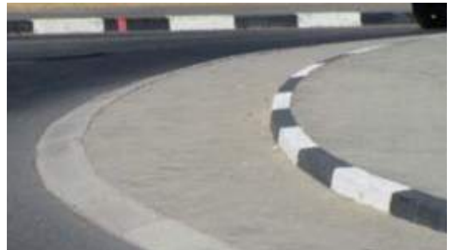
Figure 6.38: Truck apron not serving the purpose of design in South Africa (too high apron to ride on for larger trucks and too low to block riding on passenger cars).
