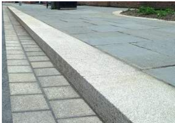
Figure 5.153: Vertical curb adjacent to footpath.
