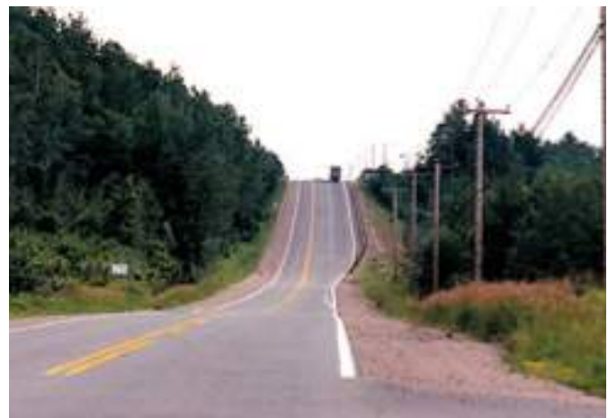
Figure 5.56: Example of markings on a climbing lane.
