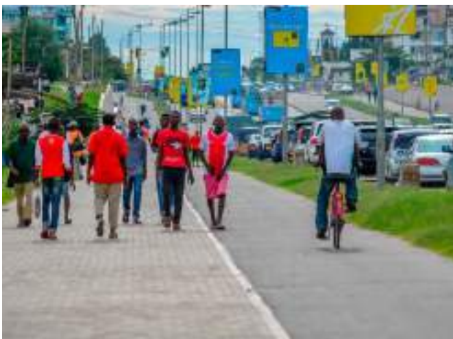
Figure 4.1: Separation of a vehicular travel way, cyclist path, and walkway on an urban arterial with concrete paving blocks on walkway and sealed cyclist path.
