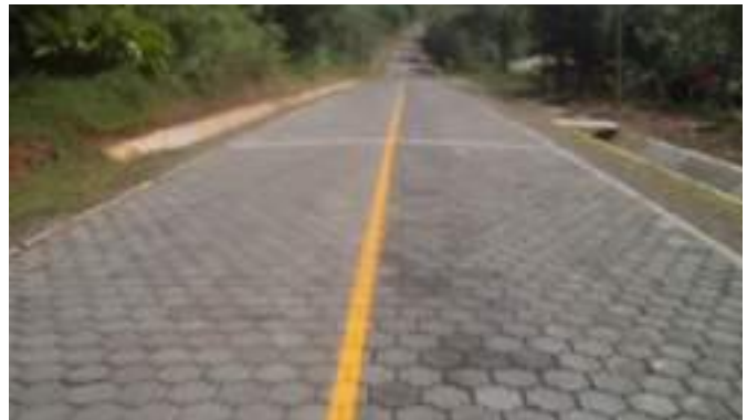
Figure 5.121: Concrete blocks (adoquines) surfacing in good condition and appropriate drainage facilities.
