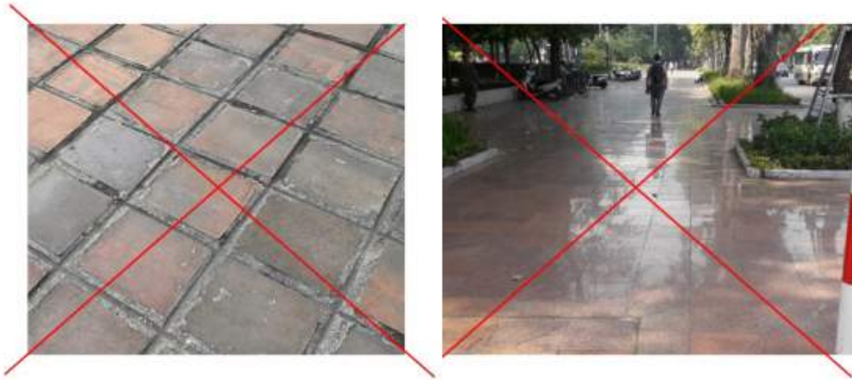
Figure 4.2: No tripping hazards or slipper floors.
