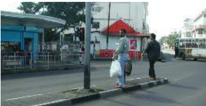
Figure 4.25: Lack of pedestrian space on median—mauritius—safety inspection.
