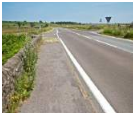
Figure 5.124: A high friction surface applied at both approaches of the intersection.
