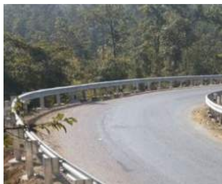
Figure 5.36: Semi-rigid barrier on horizontal curve in Nepal.
