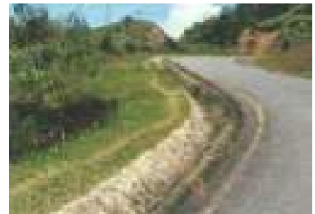
Figure 5.128: Conventional v-shaped drainage.
