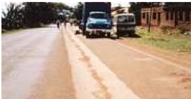
Figure 5.140: Parabolic dish drainage (good hydrodynamics but low capacity).
