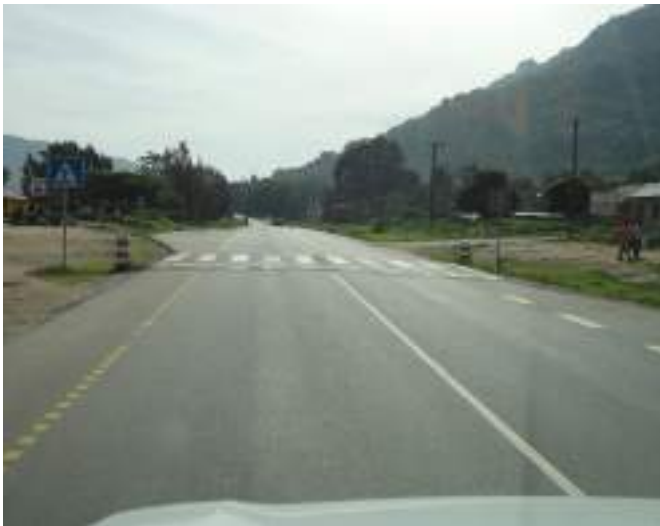
Figure 3.9: Marked speed hump for traffic calming
