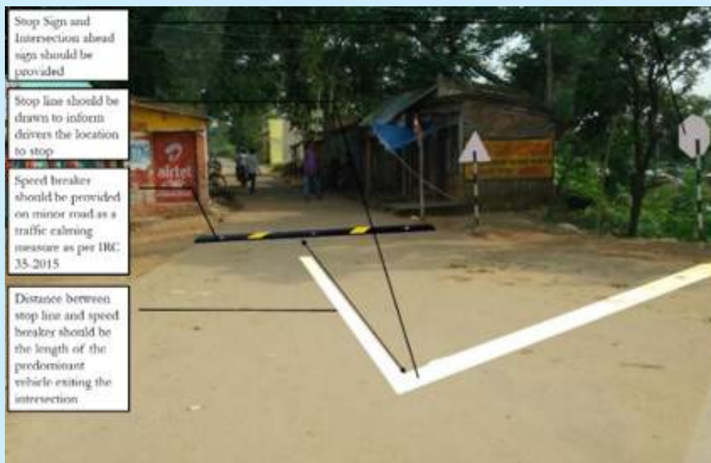
Figure 6.13: Minor road treatments—traffic calming and warning signs in India from major road perspective.
