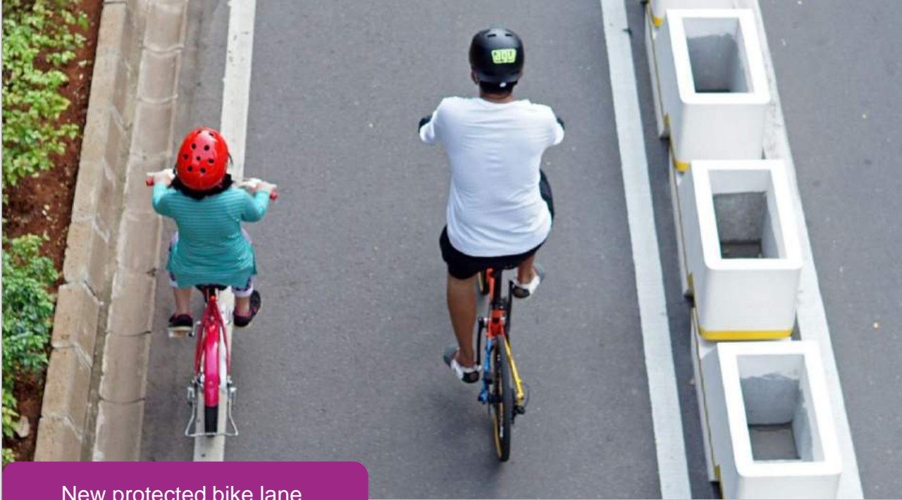
New protected bike lane in Jakarta, Indonesia
