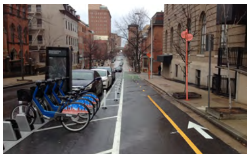
A Baltimore Bikeshare station extends the physical barrier provided by parked cars between a bike lane and vehicle traffic. Source: CharmCity123 (Flickr CC)
