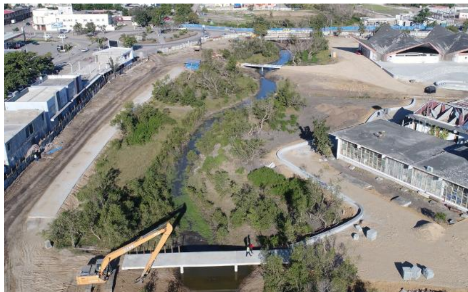
Figure 2: Chiveve Rio and Green Urban Infrastructure project during construction
